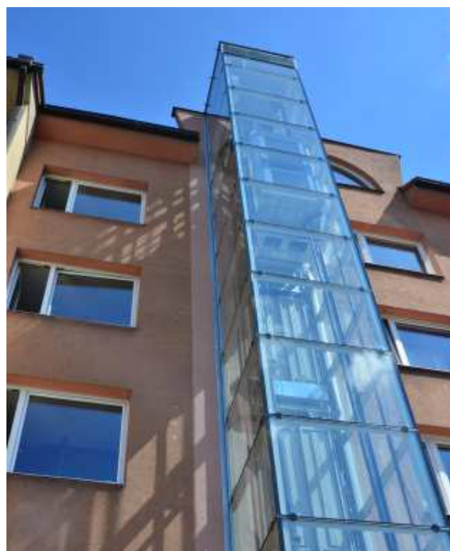
Outdoor steel elevator shaft
